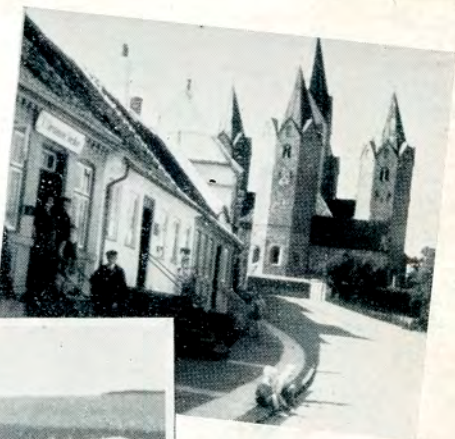
Street in Kalundborg with a glimpse of the historical church with five towers.
